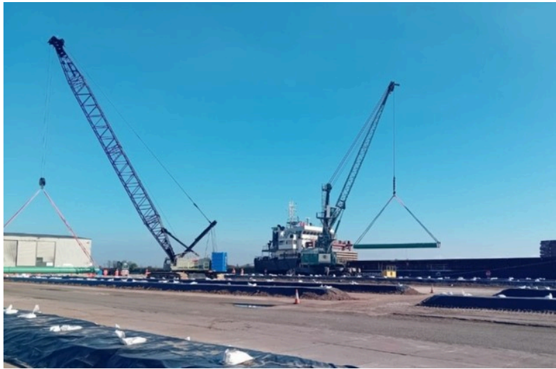
Image of Main Onshore Pipeline deliveries arriving in the UK via sea freight
